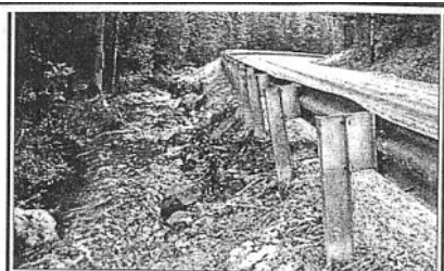
BEFORE AND AFTER—Erosion during high water flows caused the bank and road bed to drop into a brook near Scotch Hollow Road in Newbury. Reconstruction last year stabilized the bank with stone fill and realigned the brook.
